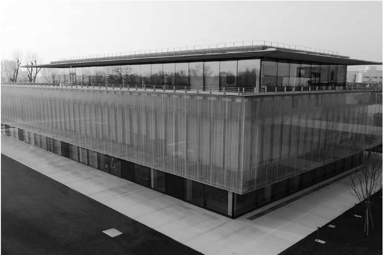
Roberto Rocca Innovation Building, a new structure dedicated to innovative teaching and transdisciplinary research.
