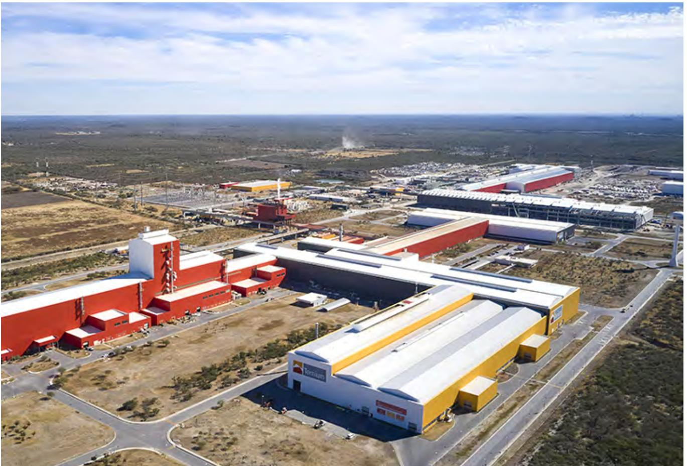
**Ternium's industrial center in Pesquería.** Upon the inauguration of the new hot-rolling mill, the industrial center will have an annual production capacity of 4.4 million tons of hot-rolled products, 1.6 million tons of cold-rolled products, 830,000 tons of hot-dipped galvanized products and 120,000 tons of pre-painted products.
