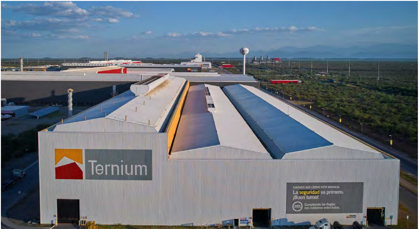
Expansion of the Pesquería Industrial Center, Mexico. Project announced with DRI-EAF technology prepared for CO 2 capture and the use of green hydrogen.
