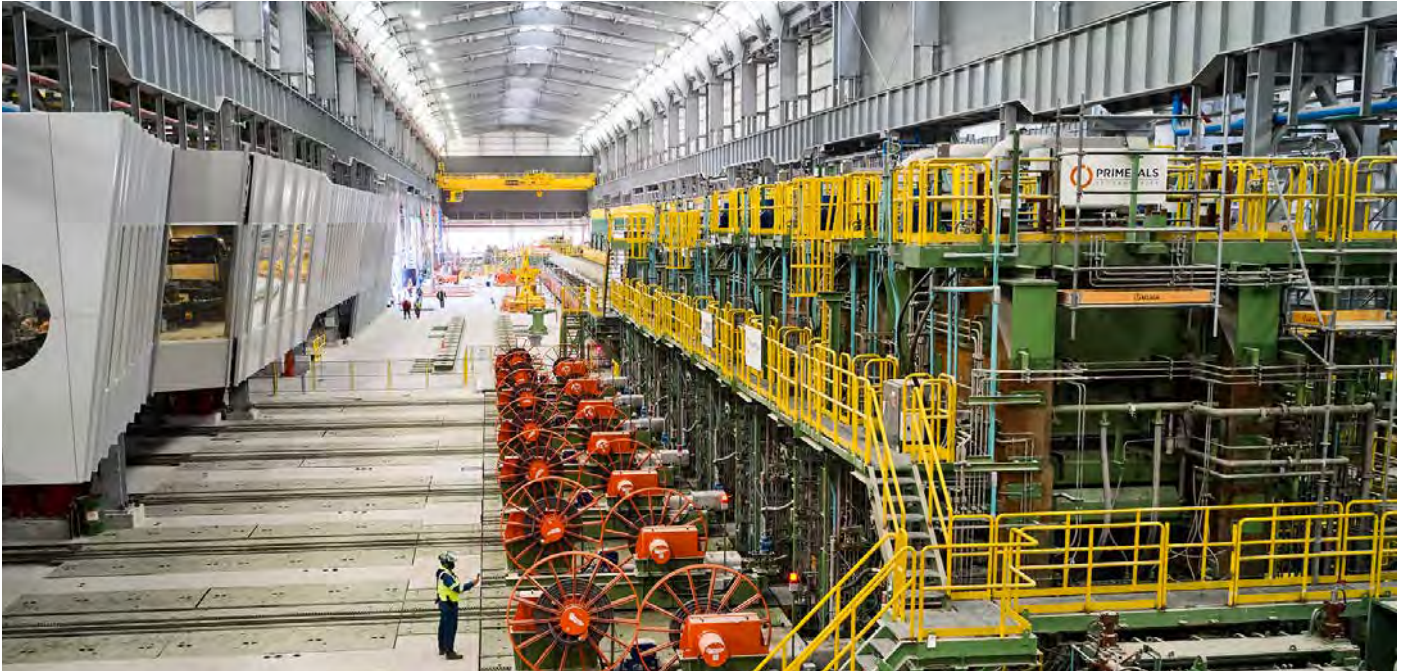
Pesquería New Hot Rolling Mill - The process of coil formation is carried out through hot rolling equipment.
